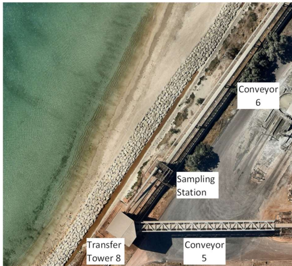
Figure 2 Completed Seawall of KBT
