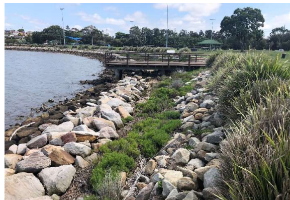
Figure 2 - Saltmarsh berms incorporated into seawall, Clayden Reserve, Sydney.
