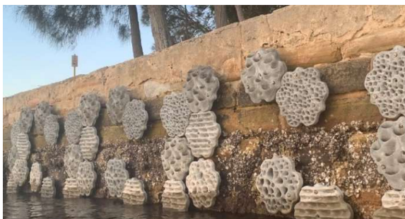
Figure 1 Living seawalls add mimics of microhabitats like rockpools that are missing from built infrastructure.
