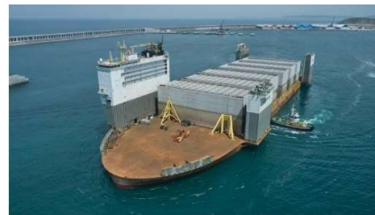
Figure 7 Installation of caissons (Source: www.puentedemando.com).
