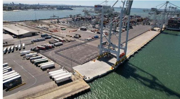
Figure 3 Webb Dock East 4 completed works, showing new cranes installed.
