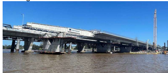
Figure 1 Photo of New Nowra Bridge during construction
