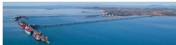
Figure 94 Approximate location of the selected jetty conveyor gallery at DBCT
