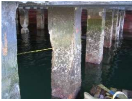
Figures 2 & 3 - (show pile conditions before and after galvanic jacket installation at North Cargo Piers
