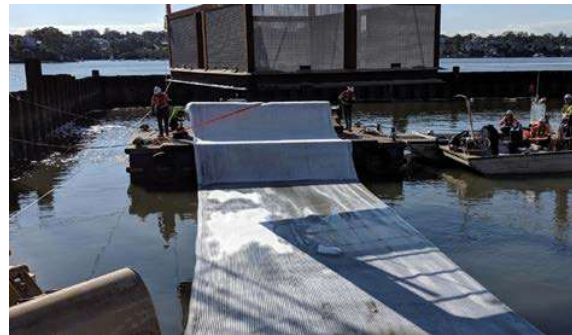
Figure 3 Ballasting of the geocomposite with a thin cobble and sand layer with the help of a sinking frame
