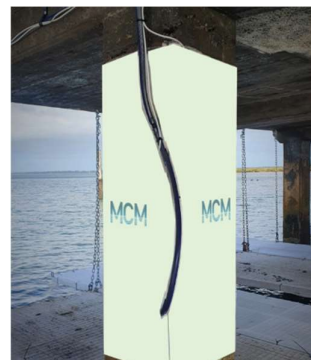
Figure 1. Typical ECE installation on a wharf pile from suspended access decks
