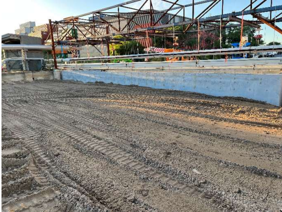
Figure 137 Permanent Culvert Completed
