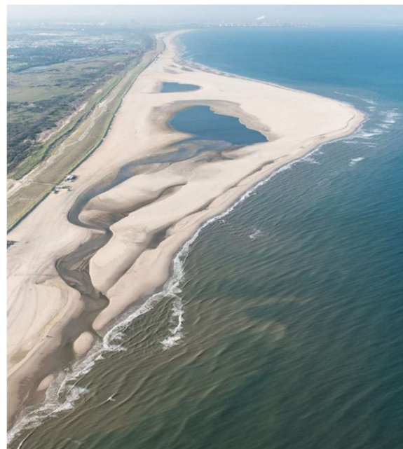
Figure 36 The Zand Motor (Source: [1]). The width of the reclamation at completion was approximately 1 km in width and 2 km in length, with an average nourishment thickness of 5 m. Note the human-made habitat lagoon in the centre of the Zand Motor
