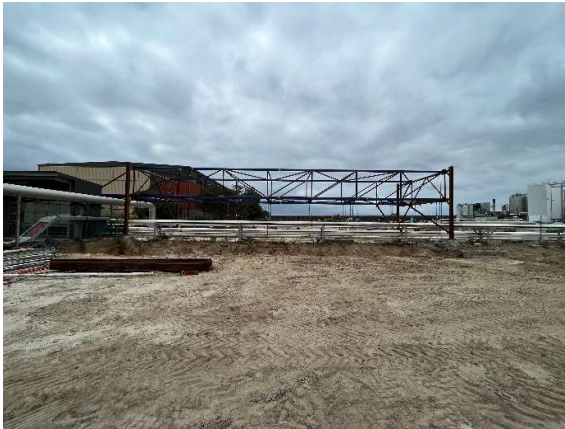
Figure 136 Temporary works structure for pipelines
