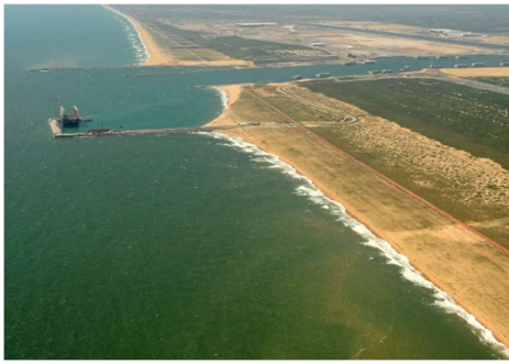
Figure 30 Auxiliary temporary port at Açú. (Source: ACCIONA).
