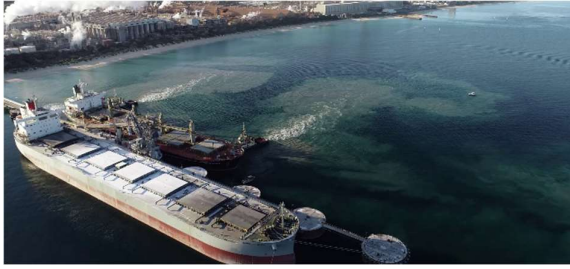
Figure 10 Alcoa Jetty during the berthing manoeuvre of KULJAK ARROW at No.2 berth (south) during the field measurement campaign, showing resuspended sediment plume due to tugs (BMT 25/08/2023).
