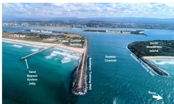
Figure 1 Gold Coast Seaway layout (Gold Coast Waterways Authority).
