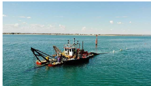
Figure 2: Dredge vessel, Ironheart, dredging Teggs Channel. Source: Maritime Constructions .
