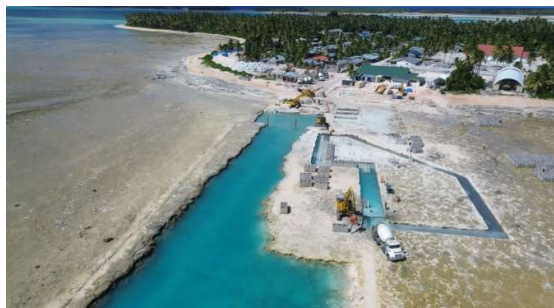
Figure 118 Small work boat harbour construction in Nui, December 2023
