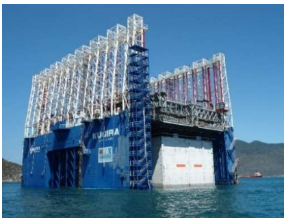
Figure 32 Fabrication with floating dock (Source: ACCIONA).
