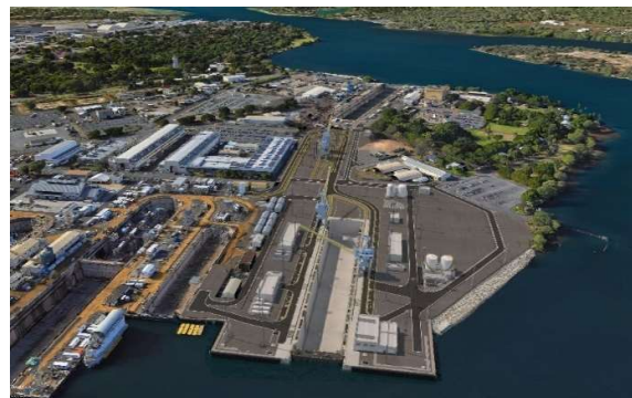
Figure 93. Rendering of New Dry Dock 5. Project. Shows graving dry dock No. 5 in forefront. This dock is capable of supporting maintenance and repair of naval vessels. Source: Moffatt & Nichol
