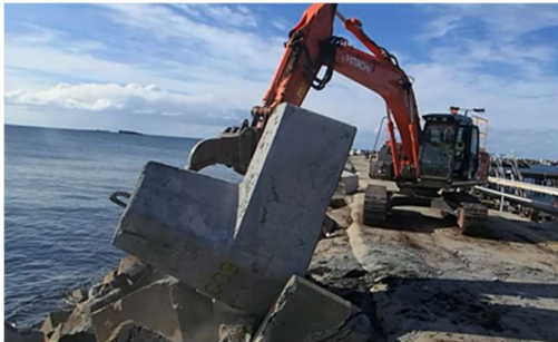
Figure 40 Placement using under-sized excavator
