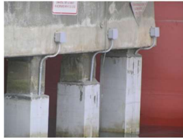
Figures 2 & 3 - (show pile conditions before and after galvanic jacket installation at North Cargo Piers
