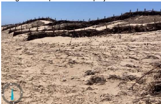
Figure 85 Drift fencing on the northern section of the dune trapping the fine particles of wind-blown sand. Source: BMT
