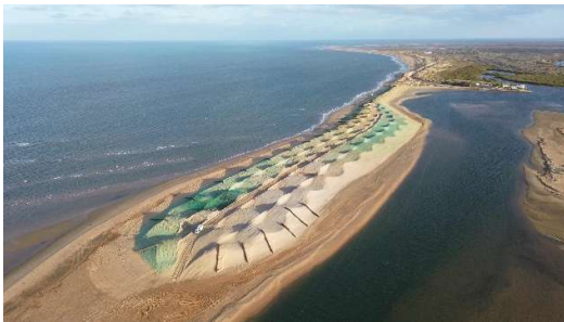
Figure 3: Stabilisation of reclaimed material Source: Maritime Constructions.
