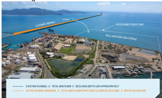
Figure 60 Channel Upgrade Project (Source: Port of Townsville)
