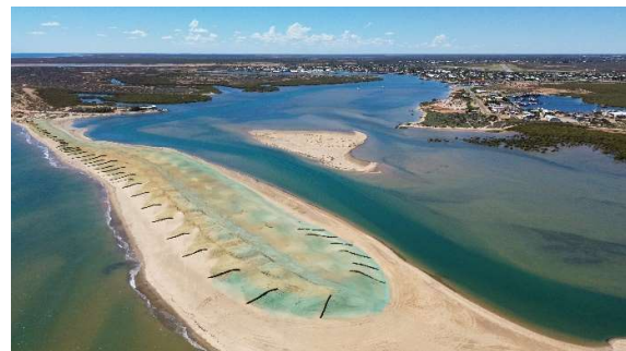
Figure 86 Completed dune construction including revegetation and stabilisation works. Source: Maritime Constructions
