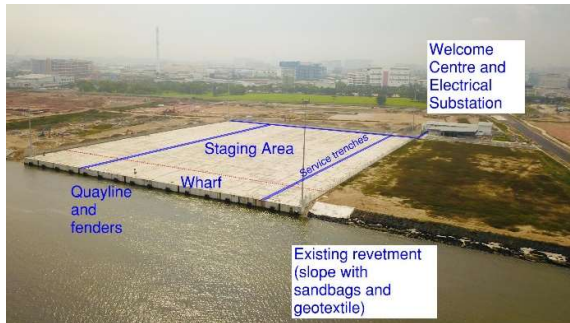
Figure 65 Site map showing major components (background photo by Penta-Ocean). Service trenches are in blue.
