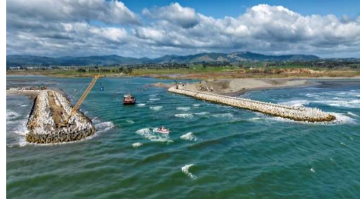
Figure 59 OHD harbour channel on its opening day [Source: ODC government]
