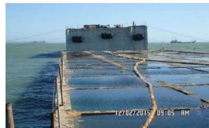
Figure 33 Installation of caissons (Source: ACCIONA).
