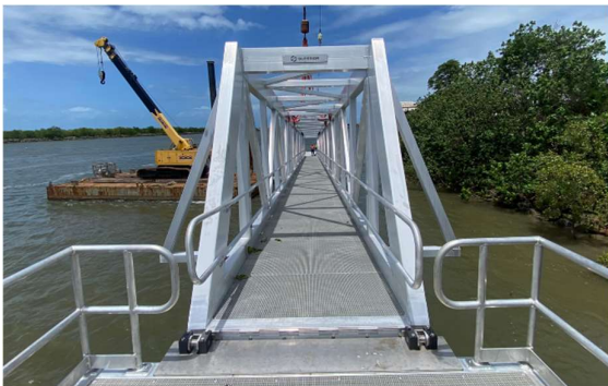
Figure 4: Gangway wishbone hanger connection to fixed platform.
