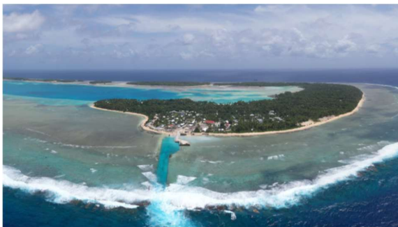
Figure 141 New excavated channel in Nui (Source: in house).
