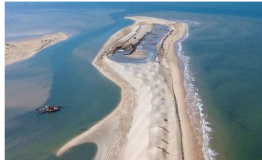
Figure 4: Progress of dune construction. Source: Maritime Constructions.
